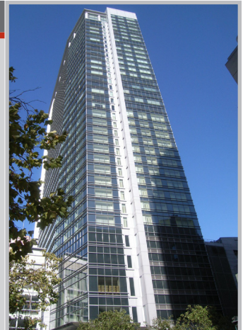
ExposureSource records contain property-specific information that describe the characteristics of a structure.
